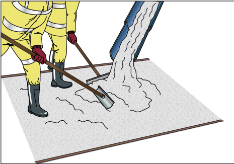
Figure 3. Concrete placing directly from the ready-mixed concrete chute.
