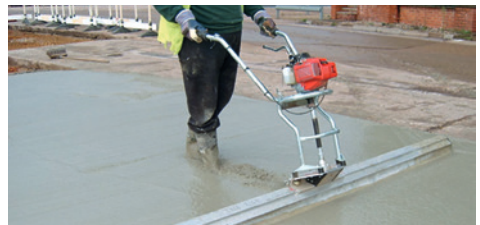
Figure 13. Petrol powered single beam screed
