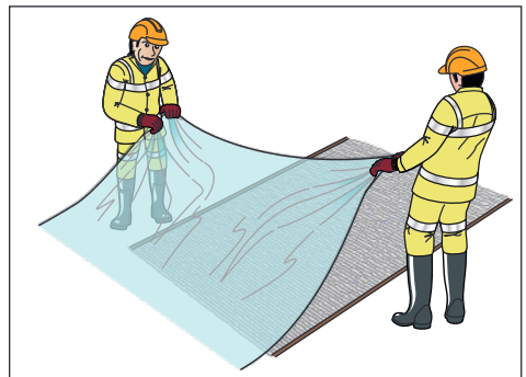
Figure 15. Polythene sheeting used to protect concrete.
